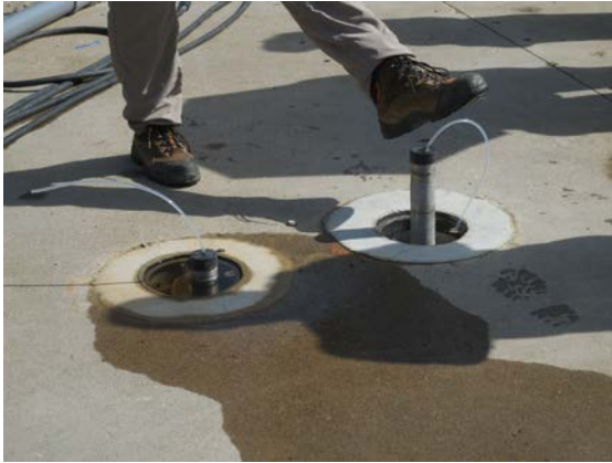
Monitoring wells completed with dedicated in-well “hot” sampling apparatus for collecting ground water samples during remediation.
